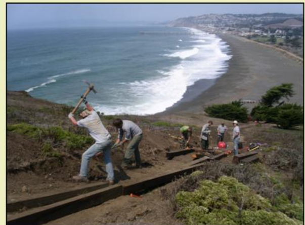
NPS Trail Crew installing timber steps
