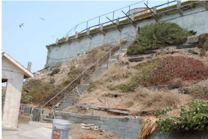
Recreation Yard Slope and retaining wall at base, summer
