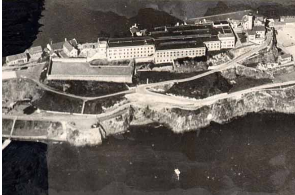
1930–1934 [SF Library], West Side, before recreation yard stairs were built
