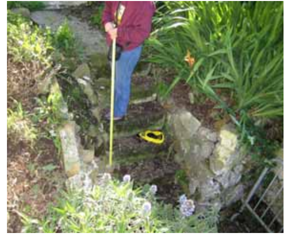
Concrete steps to toolshed from West Road
