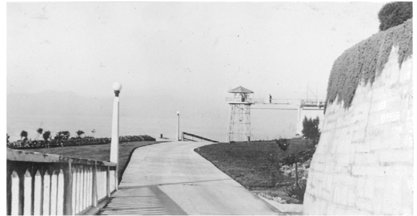
1934, West Road as it approaches the West Lawn
