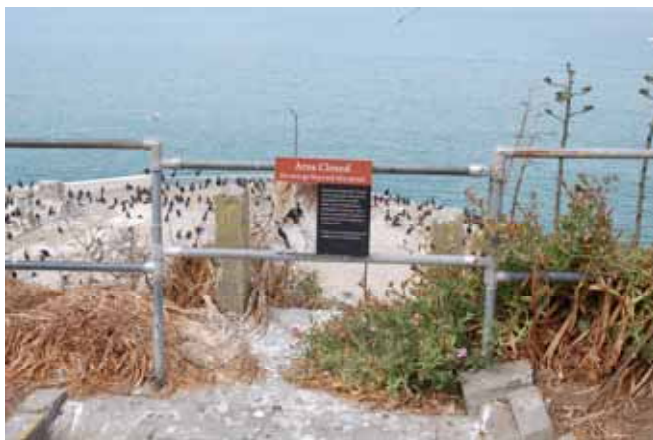
Blocked access to Laundry Terraces stairs, summer
