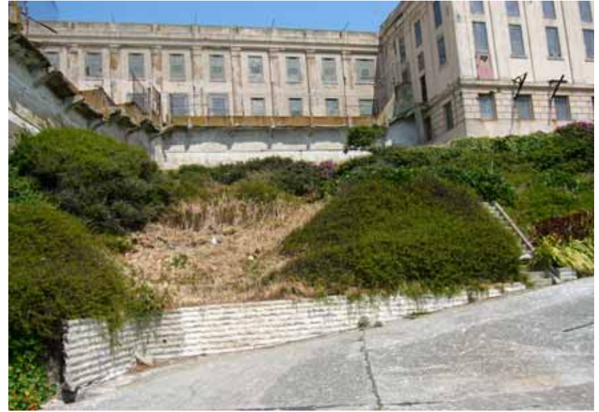
North end of West Road Terraces, showing retaining wall, summer
