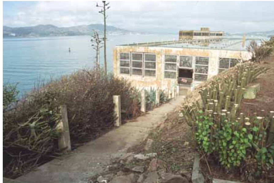
Walkway to the New Industries Building, summer
